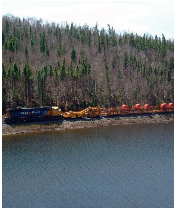
Ontera's rail plough in action
